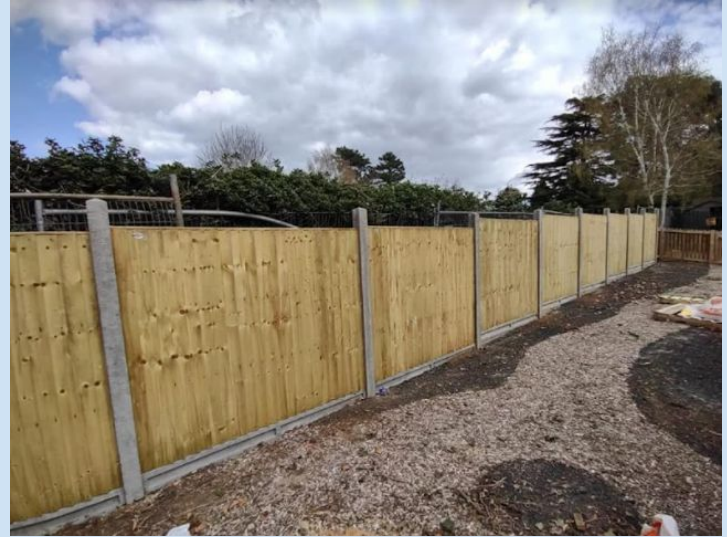
Built a fence
